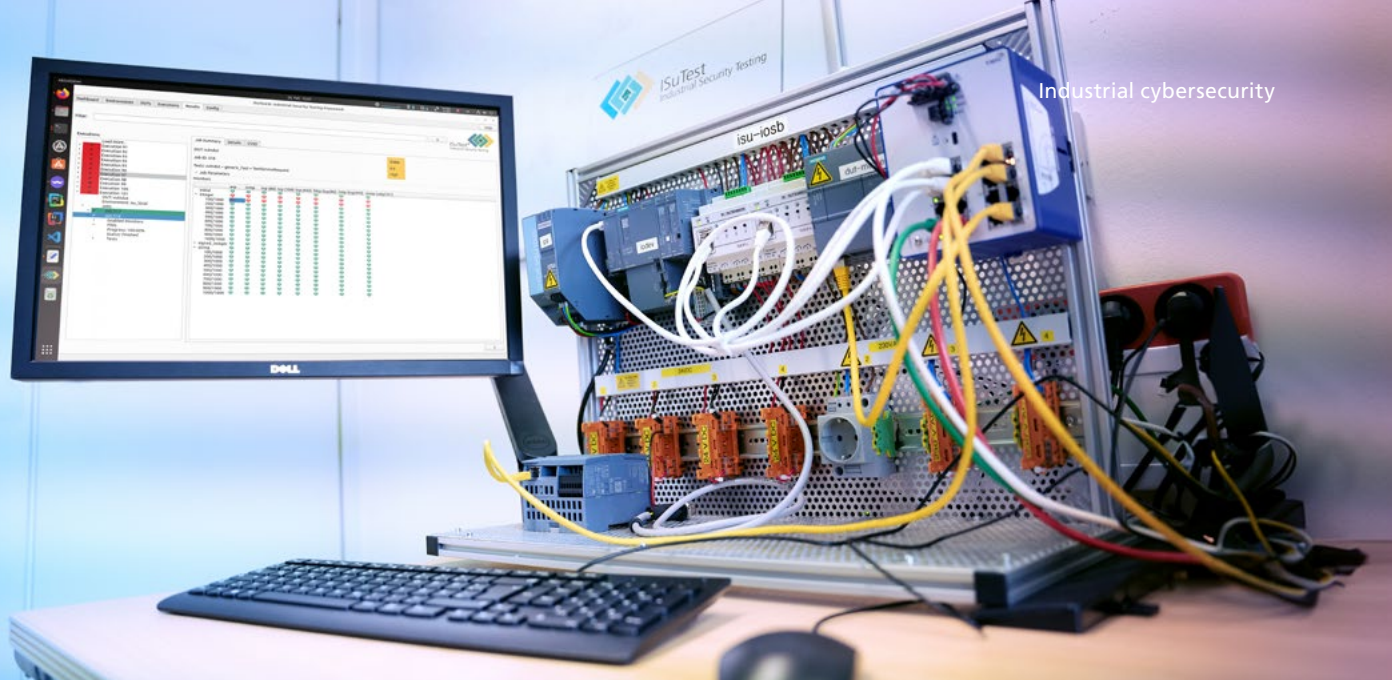
Fig. 2: Test setup of ISuTest® in the Fraunhofer IOSB laboratory in Karlsruhe.
