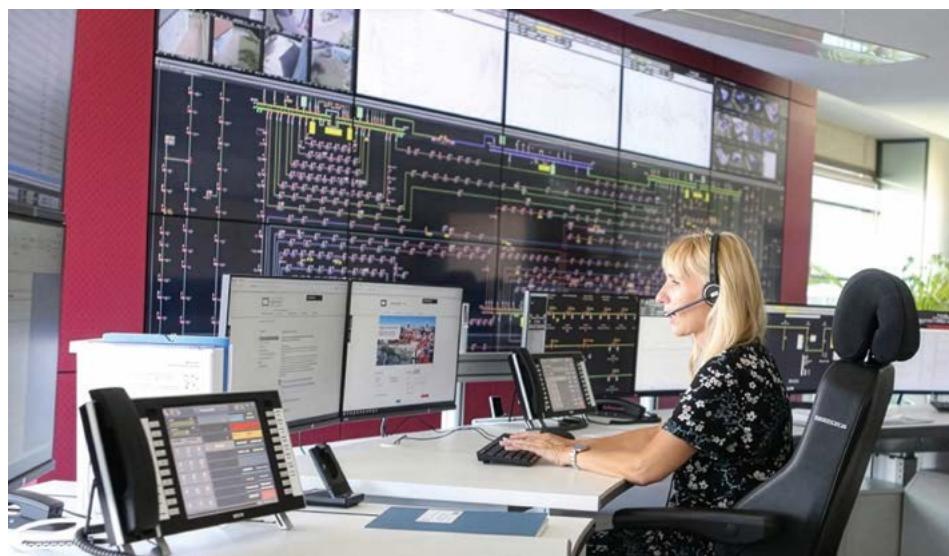
Better grid load forecasting helps minimize economic risks: inside the digital control center of SWE Netz GmbH Erfurt.
