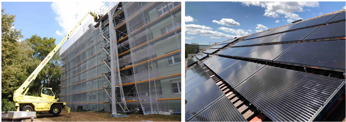
Fig. 6: Transport of SOLINK collectors to the roof of the apartment building (left). SOLINK collectors installed on the roof (one half of the roof and one half of the field) (right)
