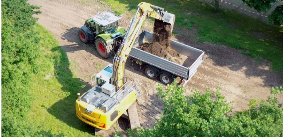
The autonomous excavator ALICE loads a transport vehicle.
